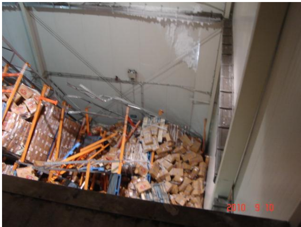
No.17 Wall pounding from collapsed racking.
