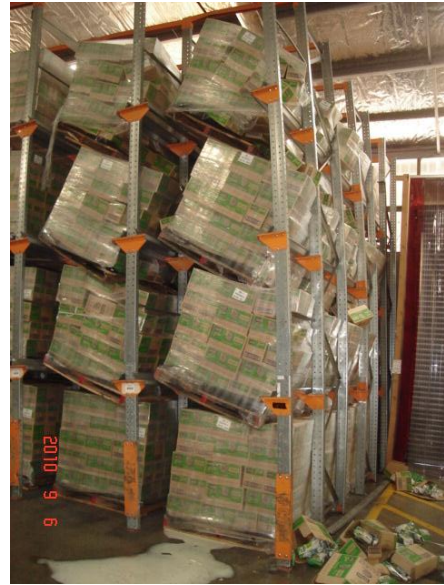
No.4 Drive-in racking.
