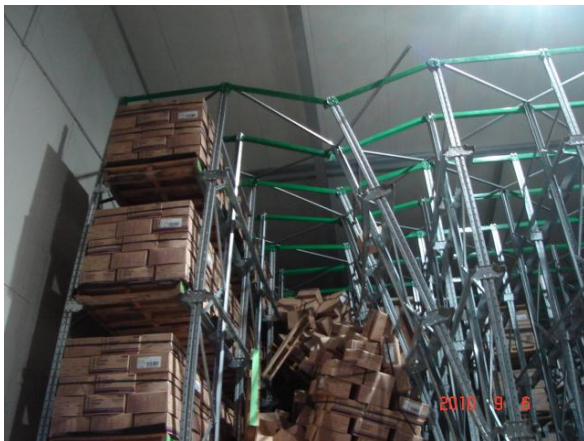
No.16 Deflected columns to drive-in racking.
