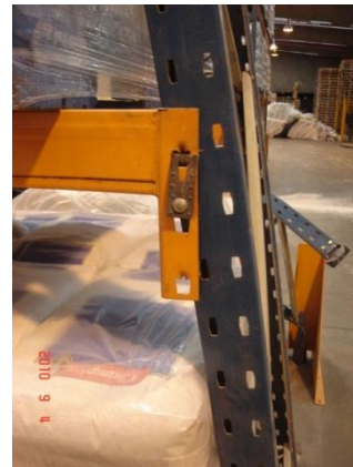
No.1 Clip beam/column joint in above.
